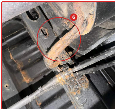
#6 Exhaust hanger and line brackets: severe corrosion
