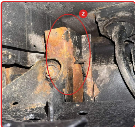
#2 Cab mount bracket: heavy scaling and delaminating metal
